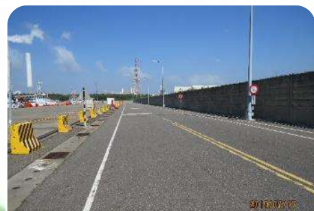
After improvement work
