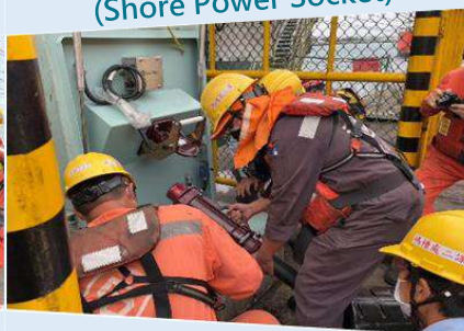
Inserting the safety locking pins
