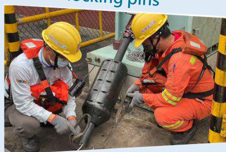
Inserting the safety locking pins
