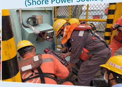
Inserting the safety locking pins
