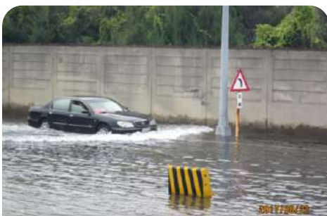
Before improvement work
